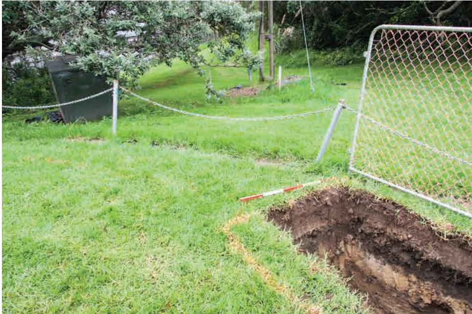
2 (left). Excavation hole for underground drilling entry point at uphill point by the new transformer location, Hapimana Street, view north.
